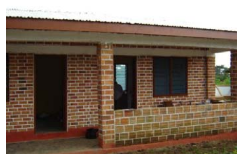
New processing plant
